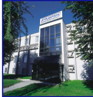
Fluiten Headquarter in Pero (Milan - Italy)
